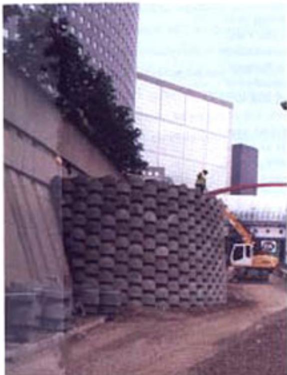
Photo 2 Raccordement au mur existant Connection to the existing wall
