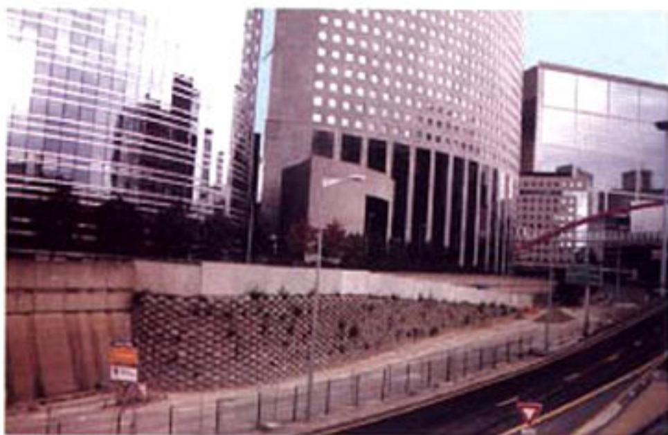
Photo 5 Vue globale de l'ouvrage fini Overall view of the finished structure
